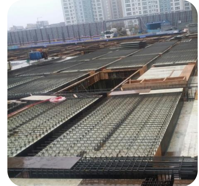
Integral Type Deck construction method
