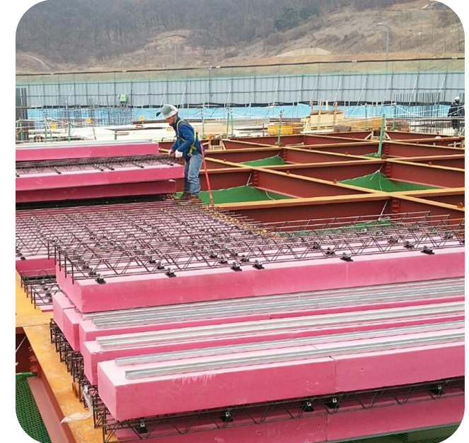
Insulation Type Deck construction method
