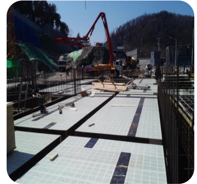
Formwork Type construction method
