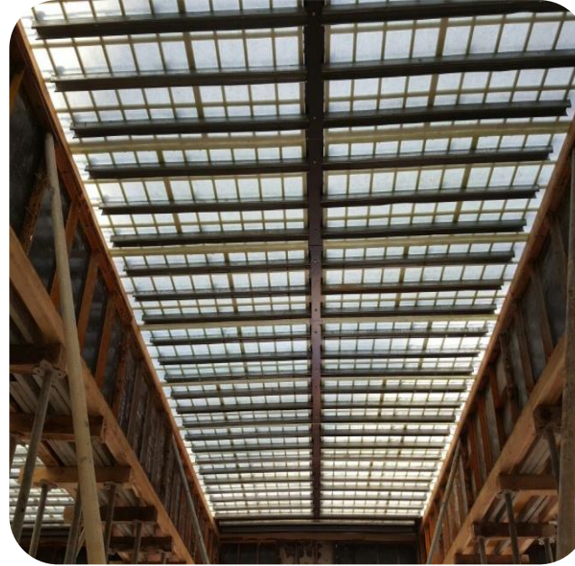
Integral Type Deck construction method
