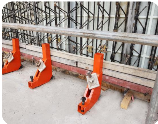
Status of fastening the bottom anchor bolt
