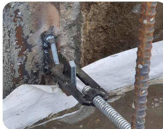
When V.H is installed separately / during precast site
