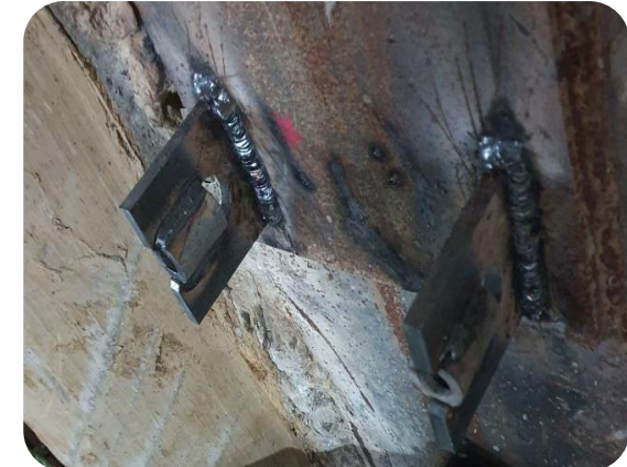
One-piece welded plate with nut / during cast-in-place site
